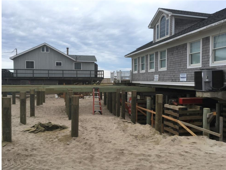
House Relocation in Dunewood - July 2017
